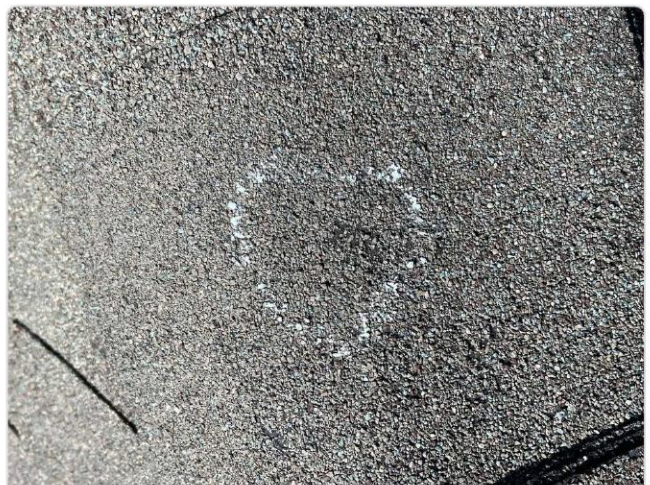
Chalk-circled hail impact on shingle surface with granule displacement — mat fracture confirmed.
