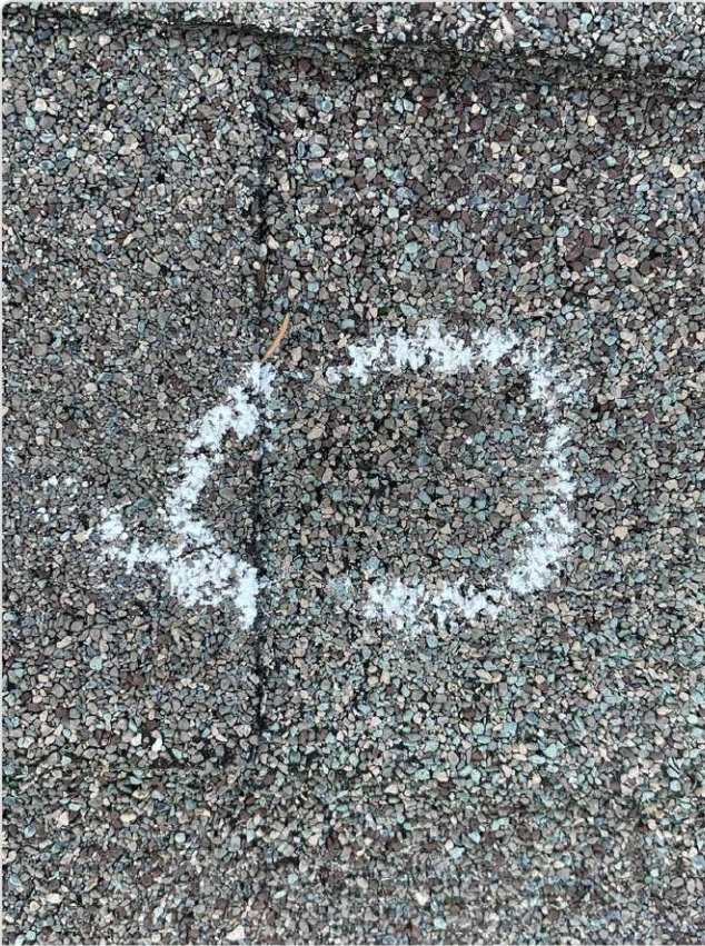
Chalk-circled hail strike on shingle shows granule loss and mat fracture at impact point.
