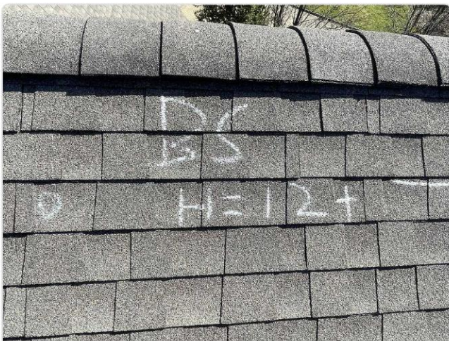
Test square markings on slope read H=12+ with chalk notation — documents hail hit density per test area.
