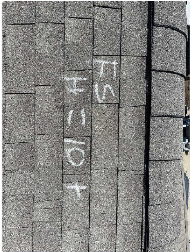
Test square marked 'TS 10+' on front slope — 10+ hail hits confirms density exceeding replacement threshold.
