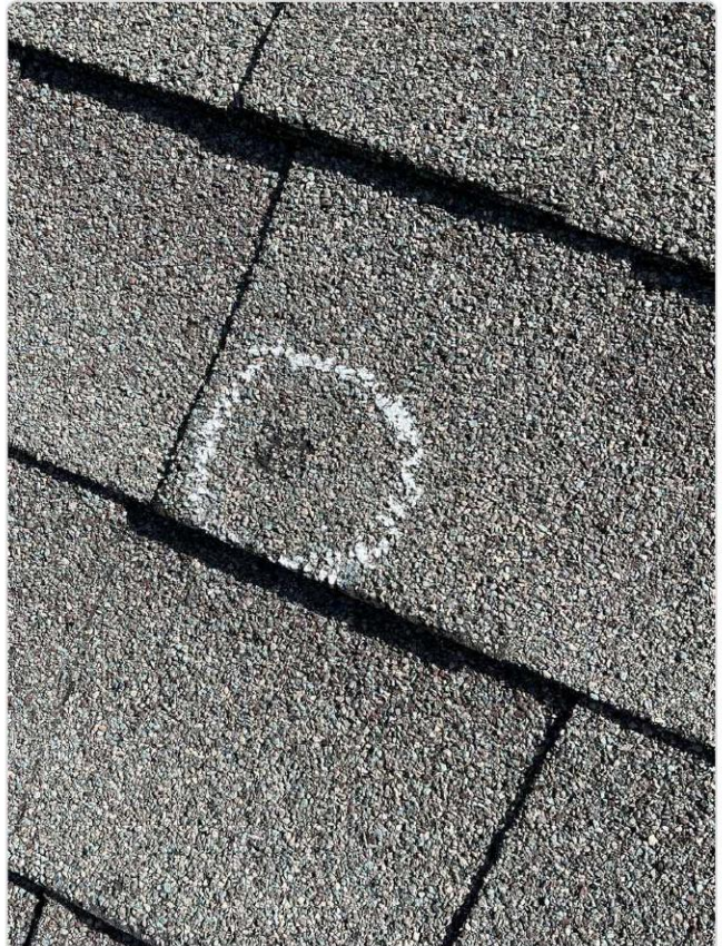
Chalk-circled hail strike on shingle shows granule displacement exposing dark mat — confirmed hail impact.
