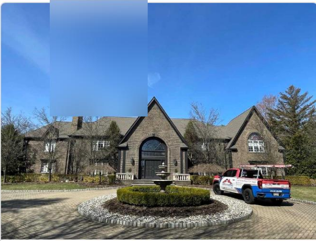
Front elevation shows large estate with steep-slope architectural shingles; roofing contractor on-site for inspection.
